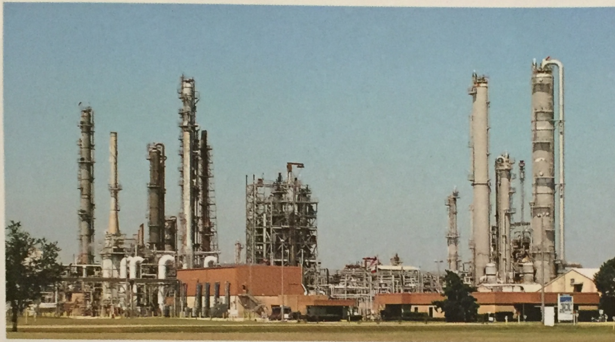
The Linde site at La Porte is expected to be commercial in January 2015.
